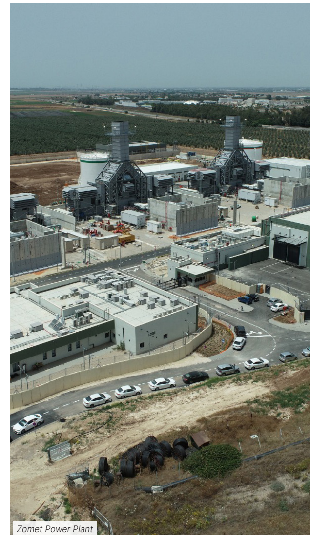
Zomet Power Plant
